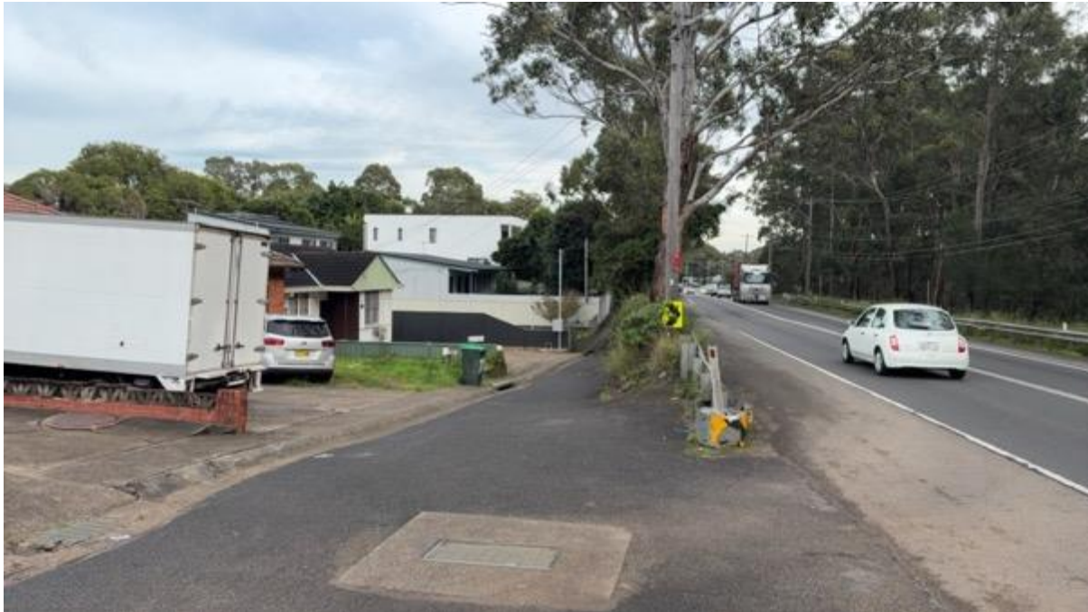
Photo 3 Indicates the small access road that connects with Henry Lawson Drive and the Woodland Classified Vegetation in the Northern aspect of the subject Lot and proposed primary dwelling in the right of the photo (Michelle Evans 2026)
